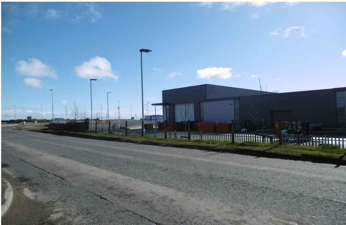
View from the appeal site to the east shows floodlights on the building opposite which are disruptive to the current residential use of the appeal site
