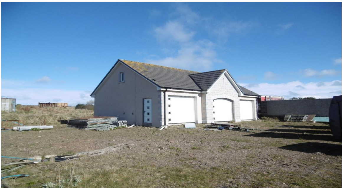
Existing triple garage to be converted to an office
